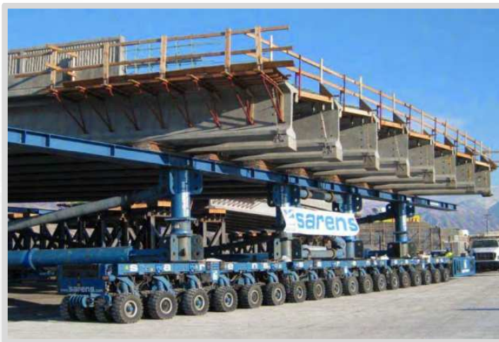
SPMT Removal/Installation
